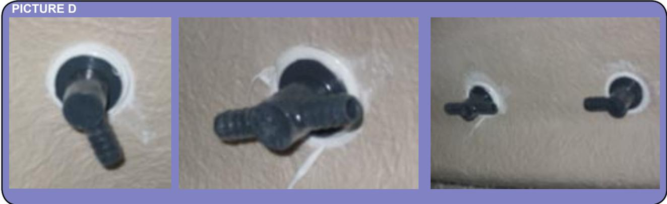
**Step 10** : if original hose is long enough to reach fitting without it being pulled tightly or causing kinks in the tubing it may be re-used, if not it must be replaced. Remember that you need to replace the lines in the same sequence and pattern as you found them.
